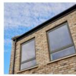
Composite windows with timber inside and powder- coated aluminium externally
